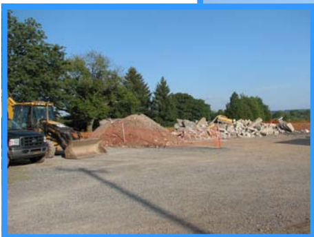
Demolition site viewed from street (Above) and rear fields (Middle)
